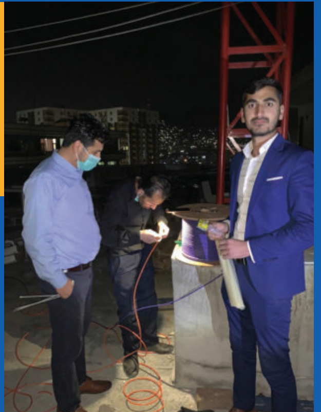
Kardan University's IT Team installing microwave devices to enhance intercampus connectivity
