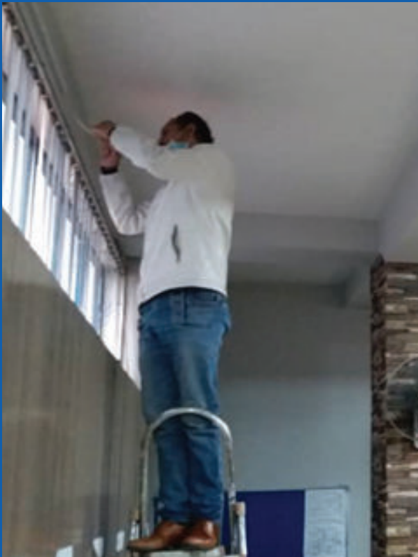
Sayed Hashmat, IT Technician, Installing New Access Points in the Faculty Room
